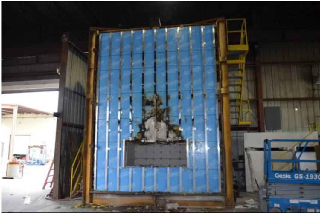
Figure C-18. Post Test Assembly Dissection – Mineral Wool Removed. Condition of Henry Blueskin following Exposure.
