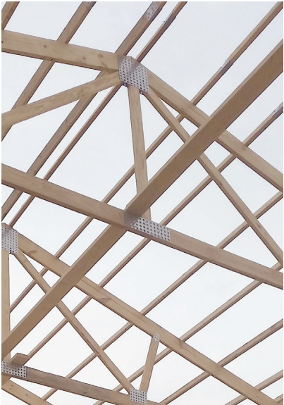
2 × 4 Purlins on end to Single Ply Roof Truss
